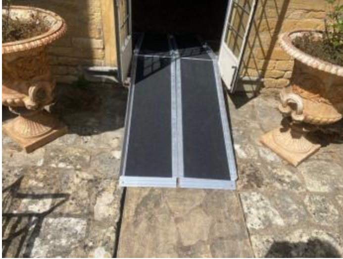
Ramp access into Museum.
