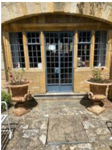
Museum can be accessed via ramp by the back door
